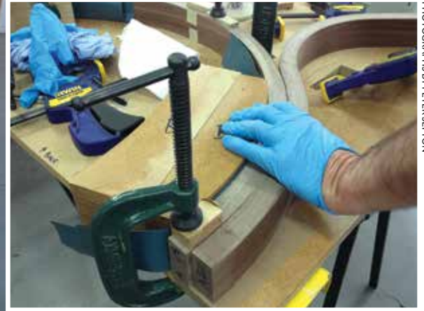
Assembly of the two matched curves on Kevan's leg frames
